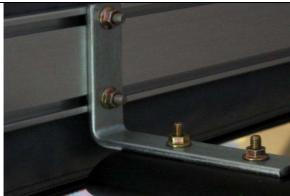
Make sure the sliding bolts have the necessary size (M6) to fit the mounting brackets. Position the brackets on top of the rack and fix them with washer, split ring and nut.
