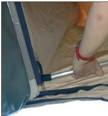
11. Retrieve the long sprung steel rods (SSR), which are positioned to tension the flysheet. Insert the bottom end of the SSR into the pre-drilled hole in the angle aluminium section, passing through the eyelet of the flysheet. This will require to bend the SSR so that the angle of the SSR is equal to the angle of the hole into which it should be inserted.
